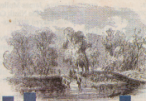
The sketch "Digging a canal across the Isthmus" is from the Civil War Harper's Weekly dated July 26, 1862. Likely sketched from a boat out in the Mississippi, the Union soldiers could be from New England, Michigan or Wisconsin.
